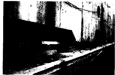
d) Hybrid isolation (sliding bearing and rubber spring)
