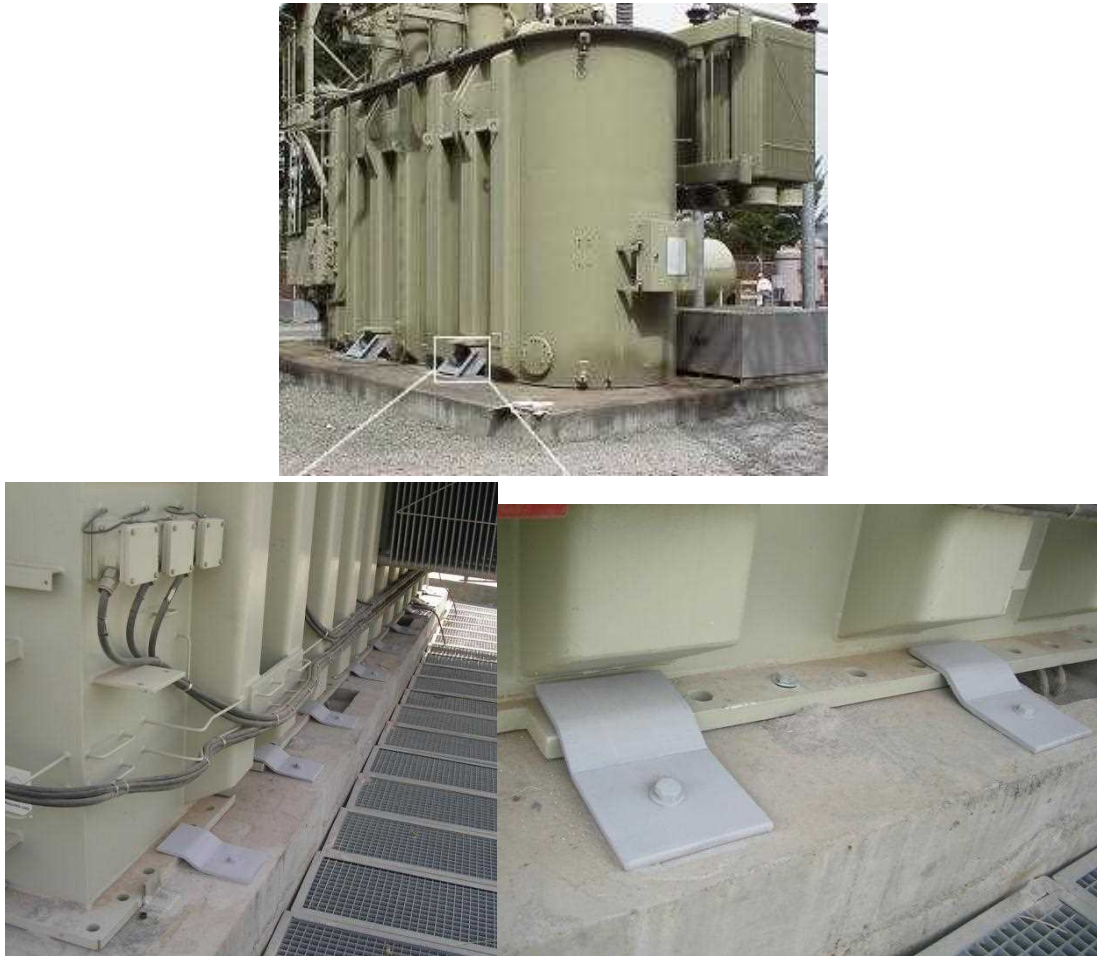
Figure 5-4: Embedding brake in transformer's leg for controlling slippage mode
