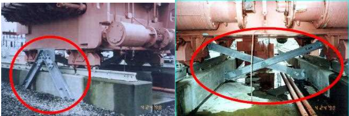
Figure 5-2: Stabilizing transformers body against overturn and slippage with bracings in leg
