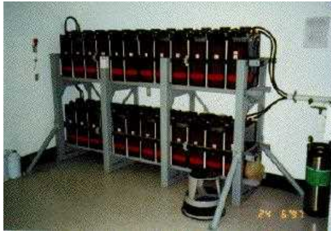
Figure 5-10: Batteries shelf bracing for controlling overturn
